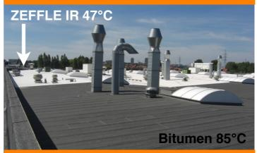
The reduced temperature of the roof, forms the foundation for effective passive cooling!
